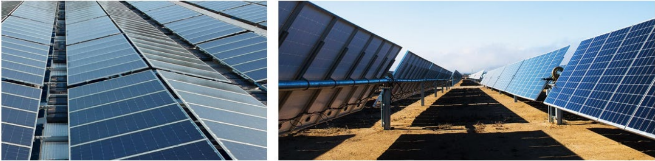
Figure 2: Fixed floating panels (BayWa r.e., left image) and active tilting ground-mount panels (NEXTracker, right image). This shows how capacity factor is a fundamental challenge for floating solar. Ground-mount panels can improve capacity factor through active tilting to follow the sun.
