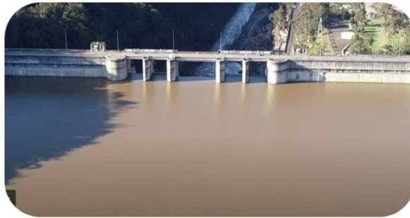
Warragamba Dam water quality degradation, post July 2022
